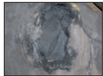
Melted or Charred areas
